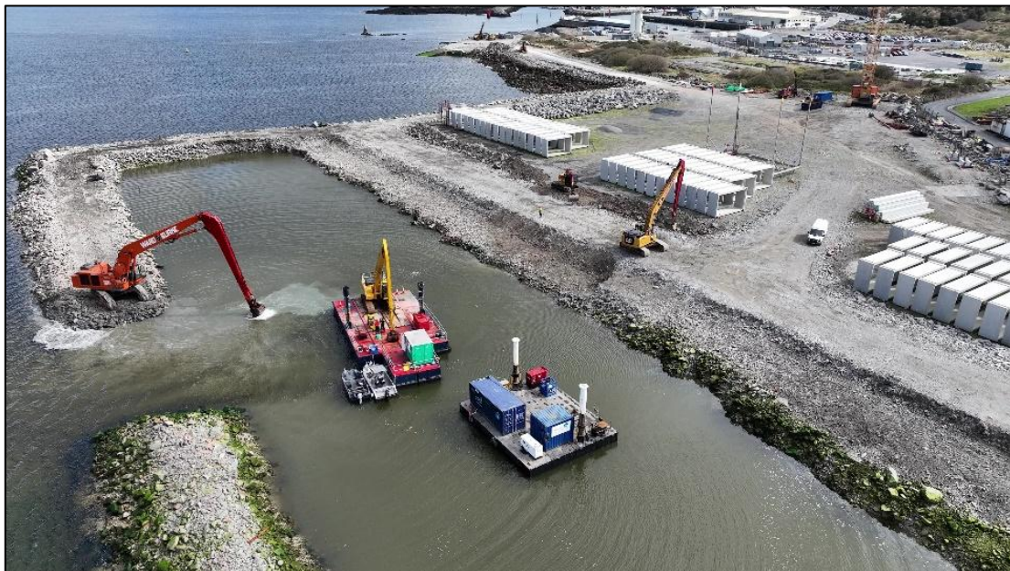
Figure 2-20: Photograph showing use of excavators on the protective berm and on floating pontoons in the constructed lagoon.
