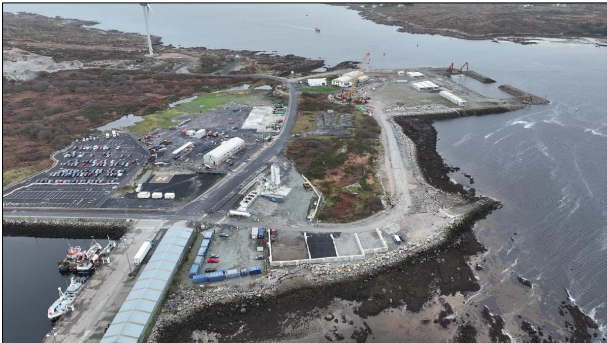
Figure 2-25: Photograph on the 14th Dec 2023 View of Compound, Concrete Batching Plant, Aggregate Storage Areas in foreground with works area in background.
