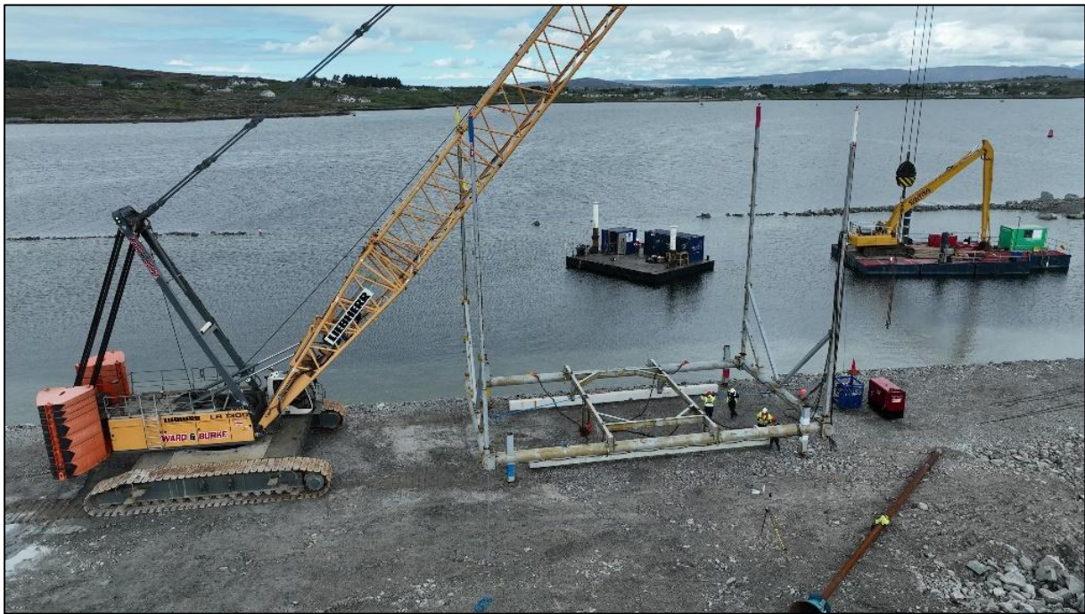
Figure 2-22: Bespoke frame used to accurately lower and position the foundation beams for the quay wall in the trench.
