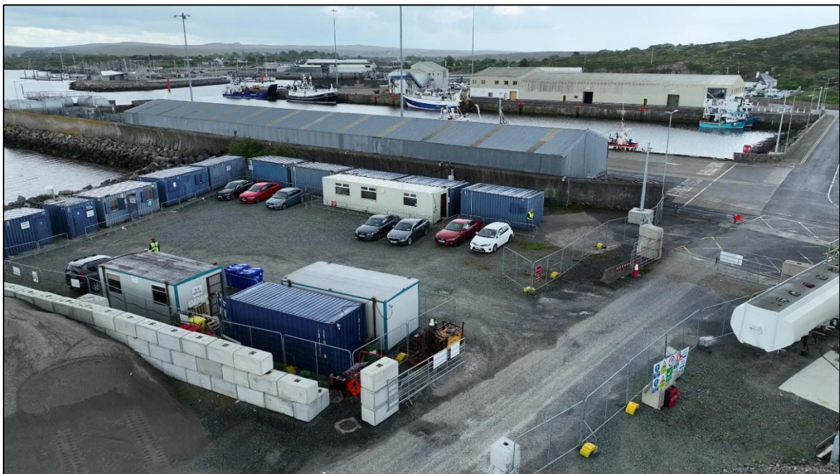
Figure 2-26: Photograph of the Construction compound with offices, storage and parking areas.
