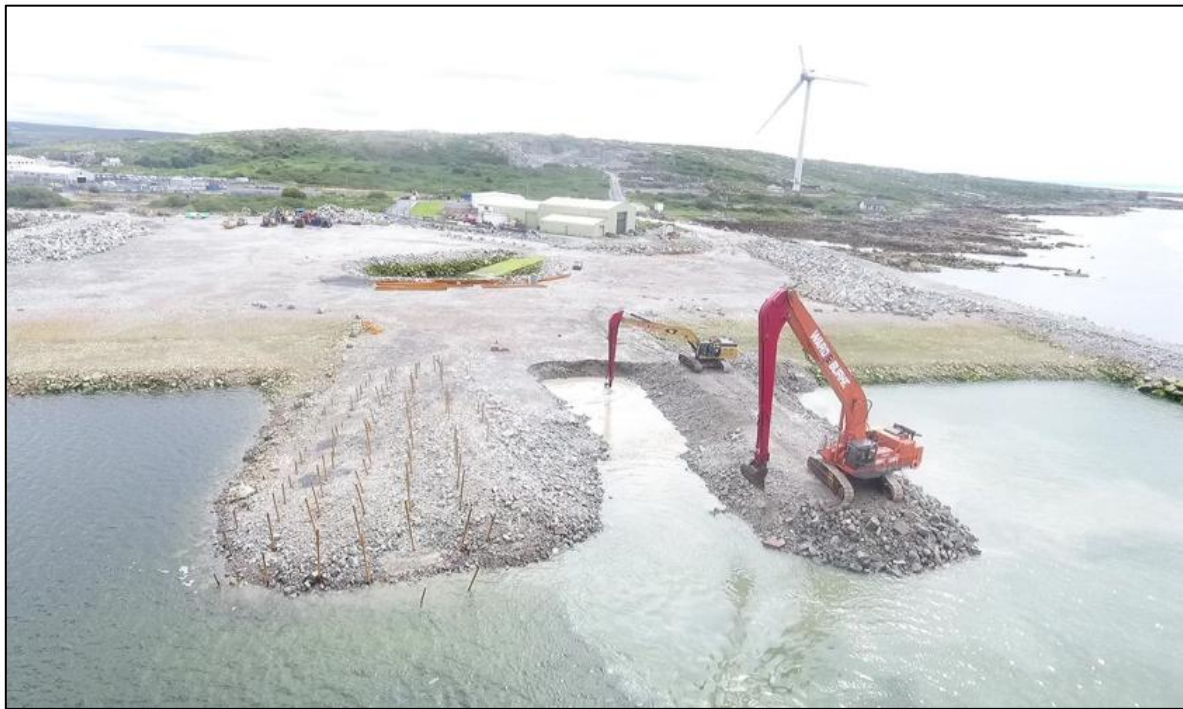
Figure 2-15: Construction of blasting platform 5 on 18th July 2023.
