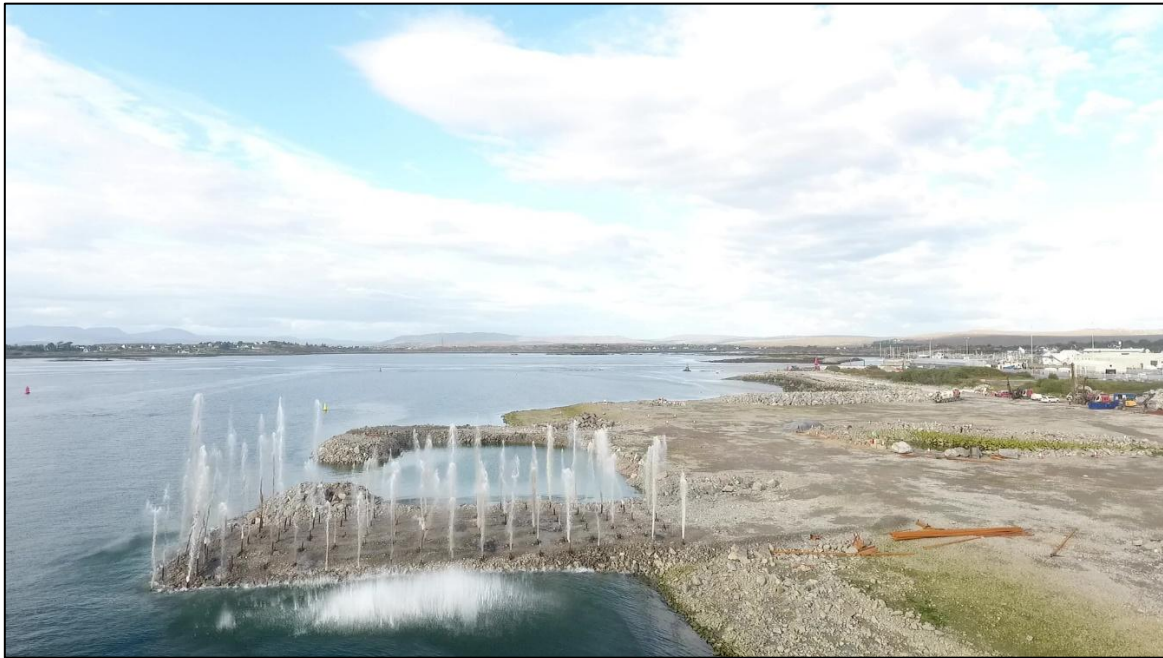
Figure 2-13: Photograph of a platform blasting event.
