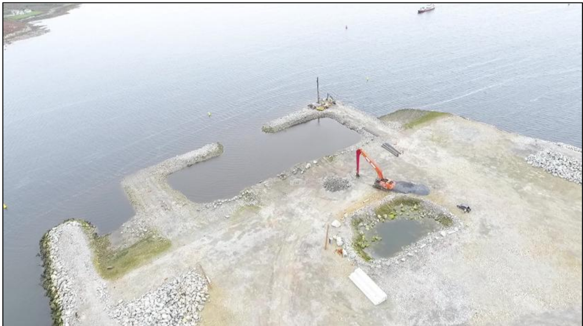
Figure 2-17: Progress with blasting platforms on 11 Oct 2023.
