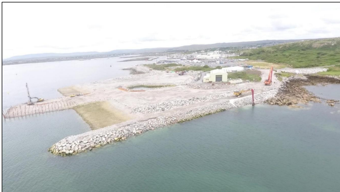
Figure 2-14: Southern protective berm with initial 3 blasting platforms in the middle of the quay wall trench on 12 July 2023.
