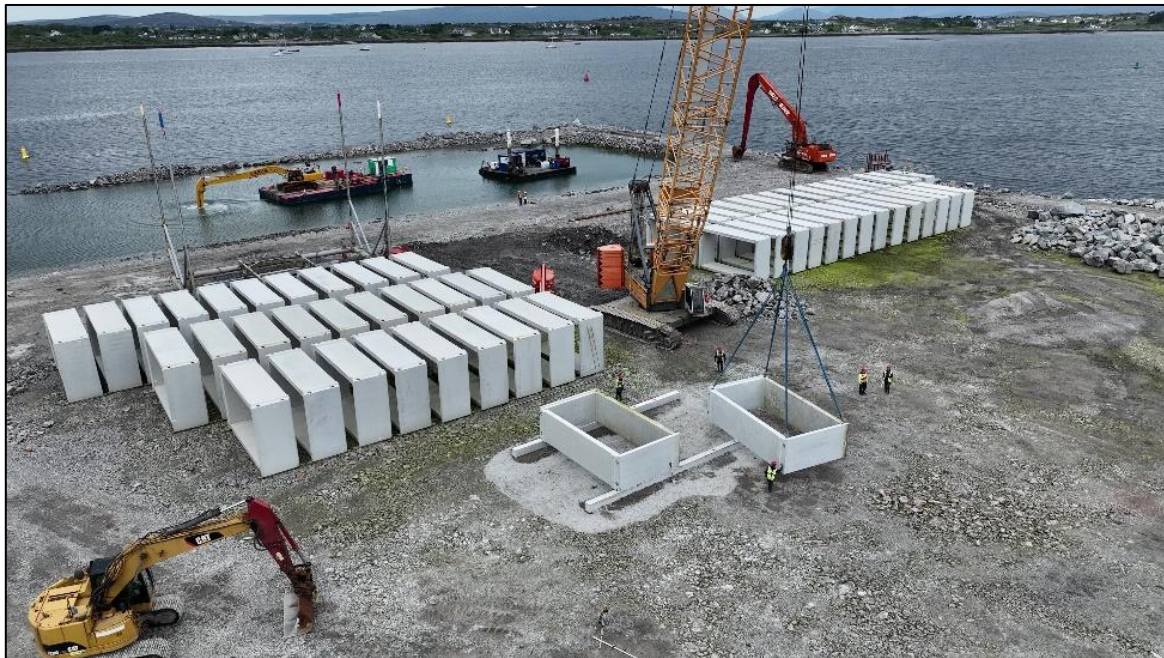
Figure 2-21: Photograph showing the (7m x 4m x 2m) concrete caisson boxes being positioned on precast concrete foundation beams positioned on the ground during a field trial on land.
