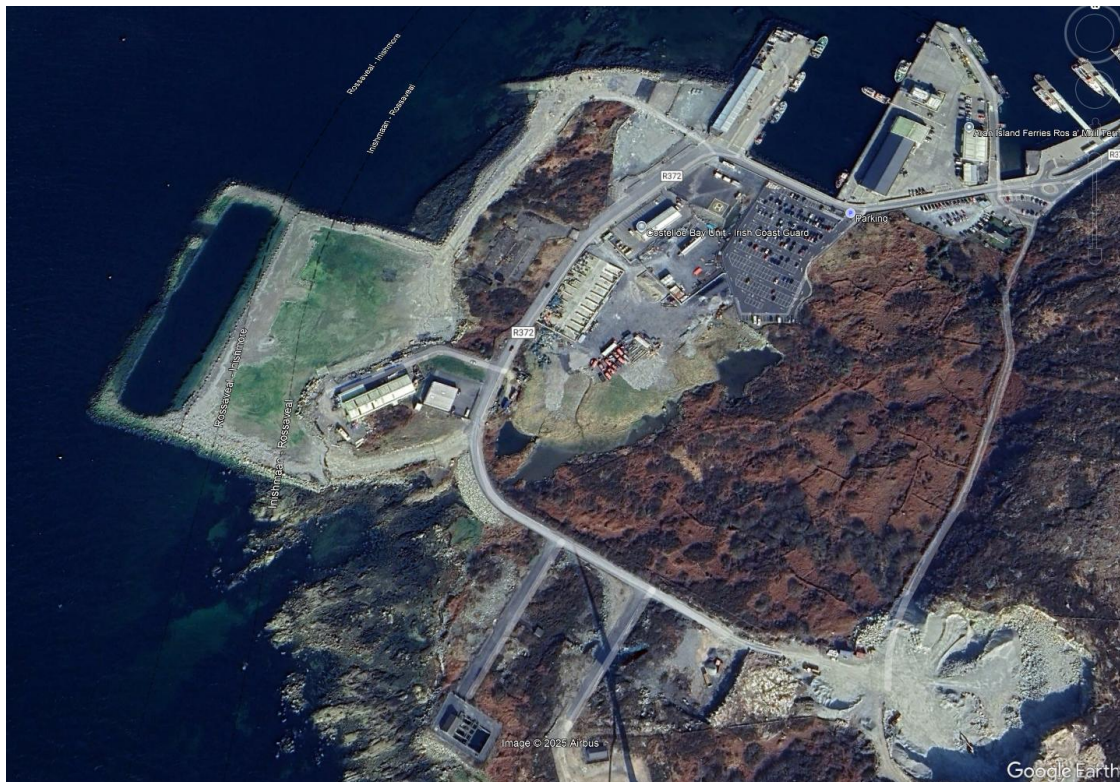
Figure 2-3 Aerial View of the development site March 2025 (Source Google Earth Pro)
