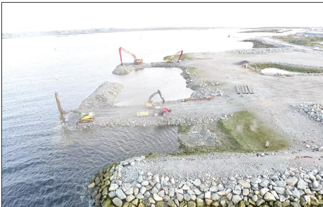
Figure 2-16: Construction of two blasting platforms on 26th Sept 2023.
