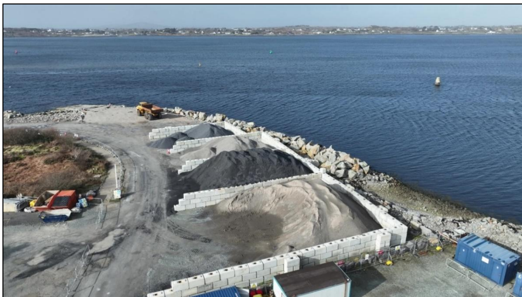
Figure 2-28: Storage areas for the construction materials and supplies for the concrete production plant adjacent to the construction compound.
