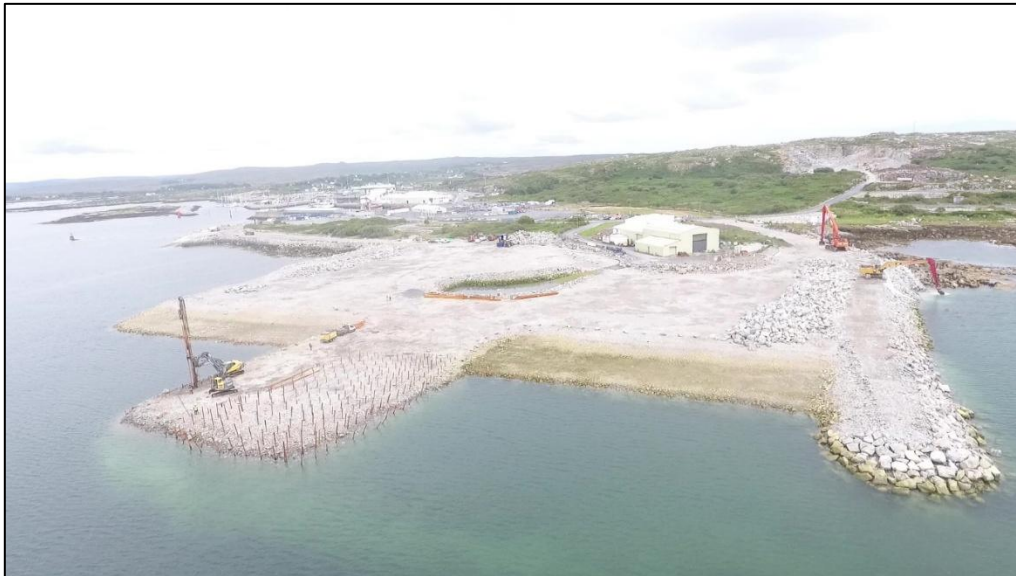
Figure 2-10: Photograph of the development site on the 10th July 2023 indicating the reclaimed area when the 2017 planning permission expired.
