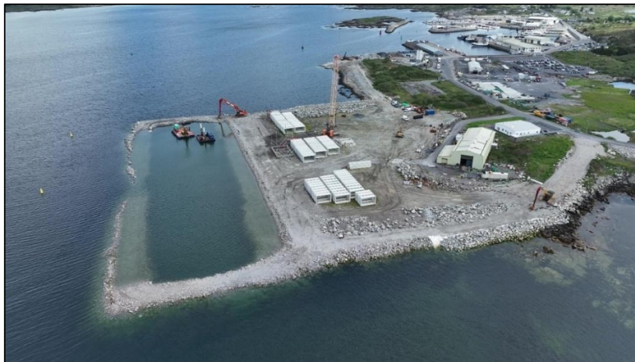
Figure 2-8: Site Status on 20 th May 2024 when the works ceased.
